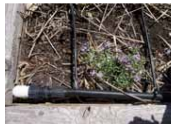
Elbow + threaded coupler + 1/2-inch tubing + 1/4-inch tubing
