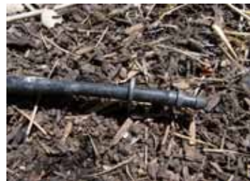
Staple securing the tubing
