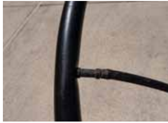
1/4-inch tubing inserted into 1/2-inch tubing
