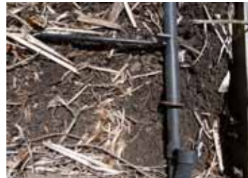
Staple securing the 1/2-inch tubing
